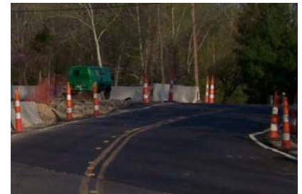
Phase 3 construction at Old 3C Highway
