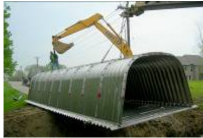
The aluminum box being lifted into place
