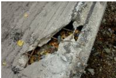
Top of concrete beam on old bridge
