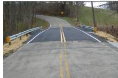
Completed bridge with new pavement
