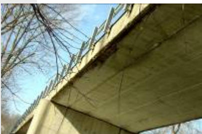
Plan to replace beams on this large bridge
