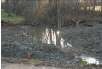
Bottom of hill where culvert will be added
