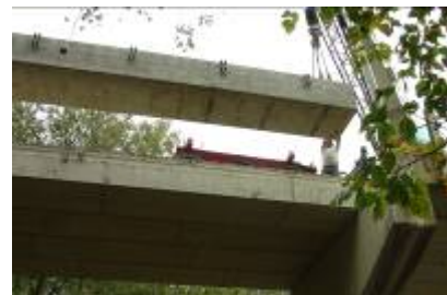
New beam being installed on bridge
