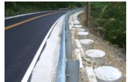
Completed pier wall
