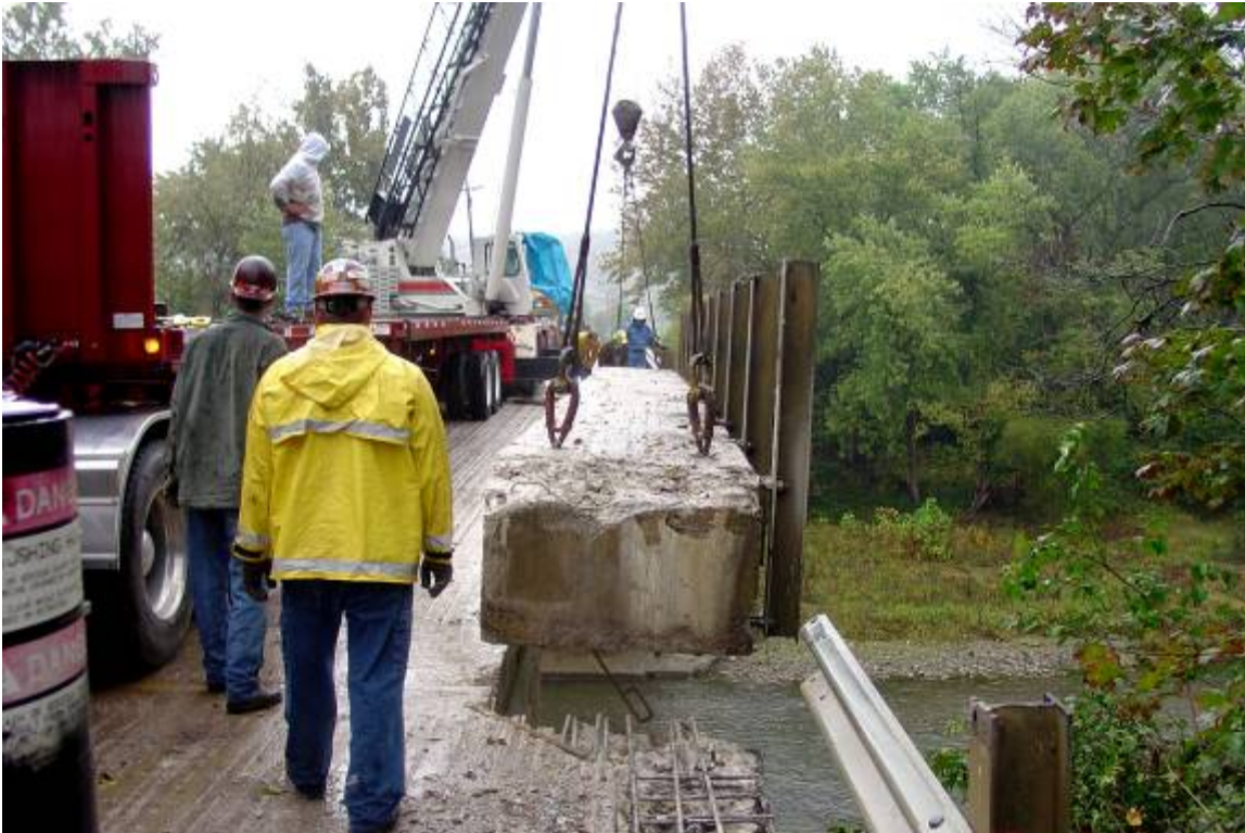
Old beam on Stubbs Mill Road Bridge being removed
