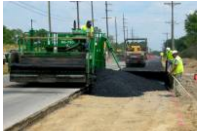
Laying the paved shoulders
