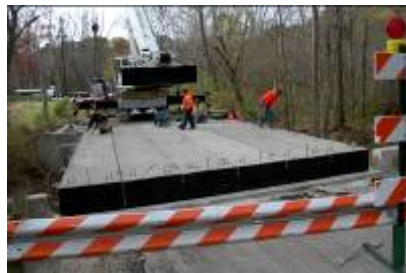
New beams being tied together
