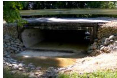
The completed new concrete box culvert
