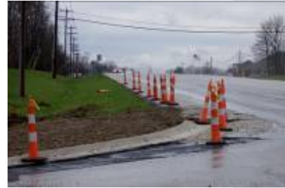
Construction improvements have begun
