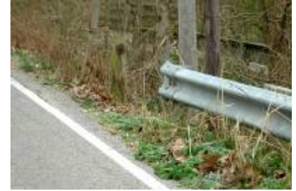
Guardrail on Corwin Road
