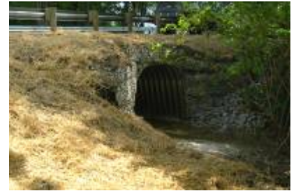
The new bridge completed
