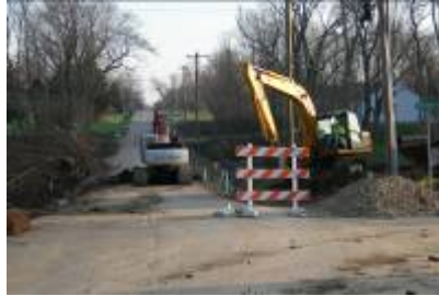
Continued construction on intersection
