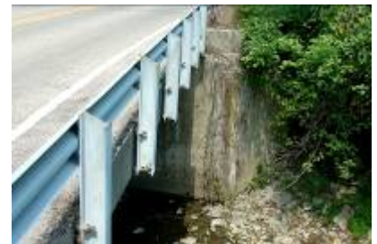
Plans are to replace this bridge's beams
